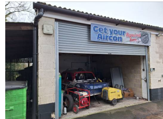
Rear Industrial Unit
