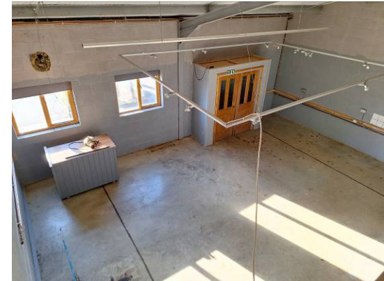
Unit 3- View from the mezzanine
